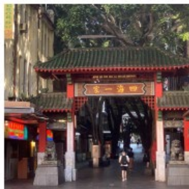
Restoration of the Gates
